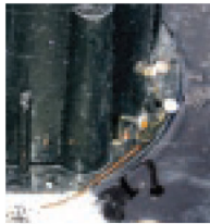
Excessive nailing
