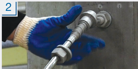
2 Remove the nut, the face washer and the spring shear sleeve and slide along the handle of the tool.
