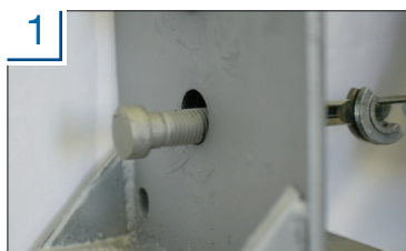
1 Install the bolt into the hole followed by the collapsible washer.
