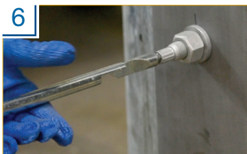
6 Remove the tool by unscrewing it from bolt (counter-clockwise).
