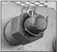
Cotter Pin Install Example
