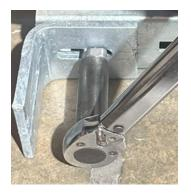
**5.** Tighten the nut to its final torque of 90 ft-lbs. Note, the T-bolt will turn to the vertical position as it is tightened.
